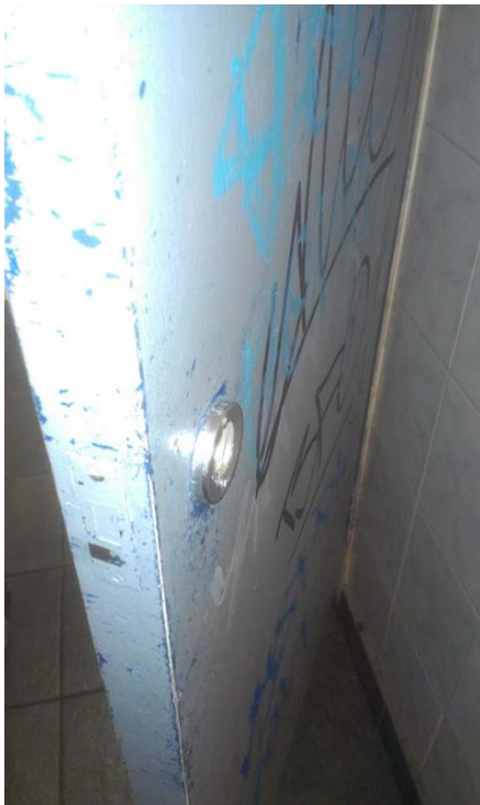
5) Poorly maintained toilet facilities- no locks or handles on doors.
