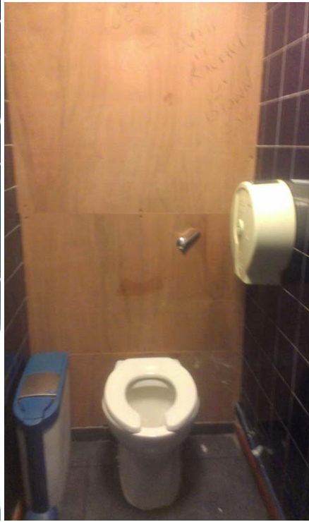
10) Water pipes loose from fixings and untreated wooden surface in toilet areas
