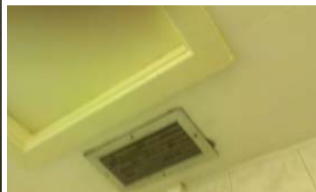
6) Poorly maintained toilet facilities-unrepaired damage and dirty ventilation.
