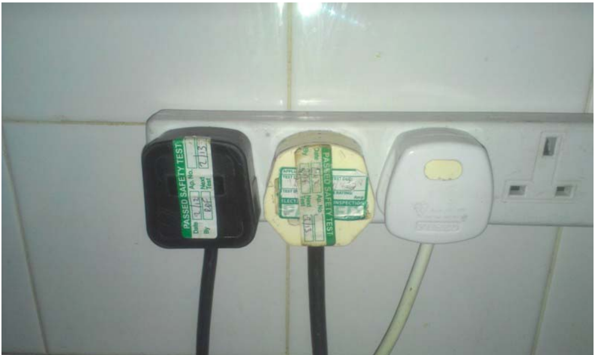
8) Unclear PAT testing system
