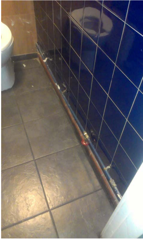
10) Water pipes loose from fixings and untreated wooden surface in toilet areas
